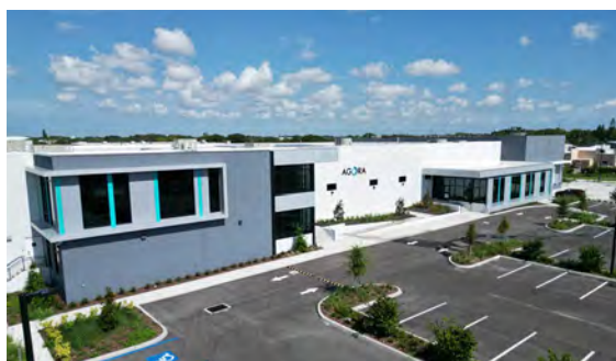
AGORA Edge ESP Completed Project
