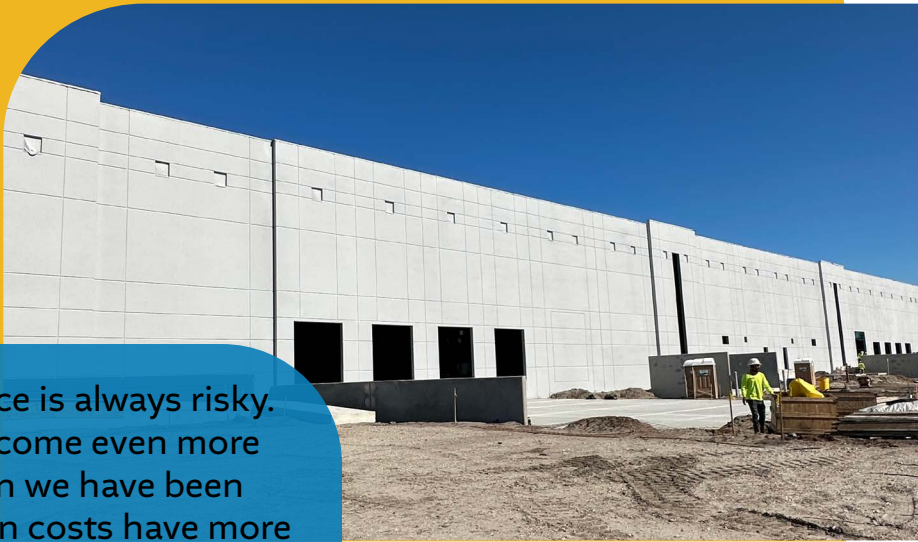
Pictured: The CMNY Transitions, LLC project features 86,350 square feet of light manufacturing space with 30-foot minimum clear height ceilings, 3 phase power, eight dock-high overhead doors, drive-in ramps and 122 parking spaces.
