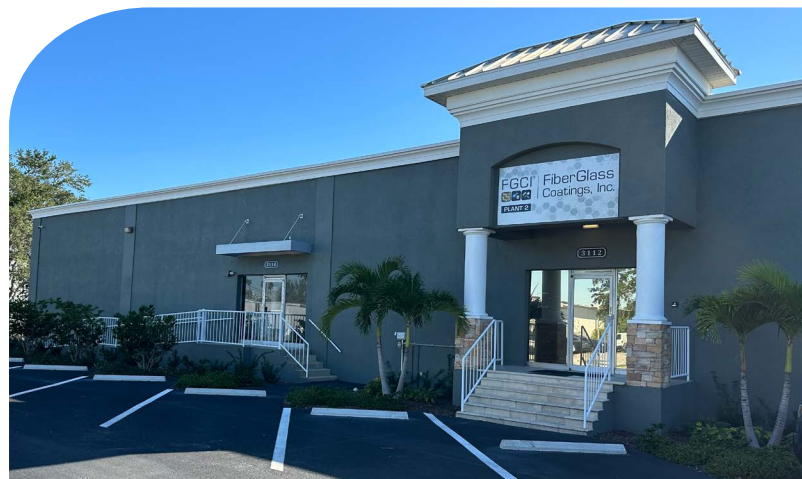
Pictured: The B&R Enterprise property is a facility that underwent a rehabilitation and renovation to 22,551 square feet of industrial space at 4301 34th St N in Lealman. The property is home to Fiberglass Coatings, Inc., a leading supplier of composite materials in the United States.
